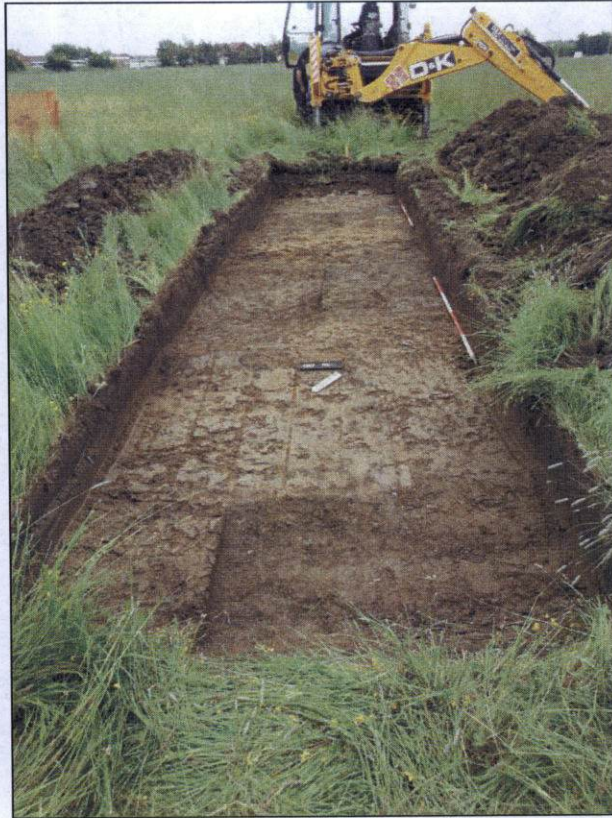
Figure 5. Trench 2 looking south east. Scales = 2 x 2m.
